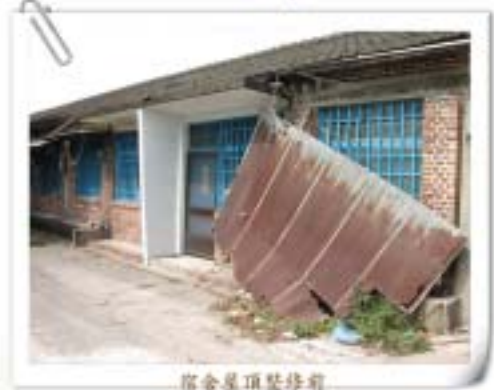
宿舍屋頂整修前
